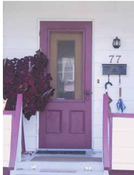
↑ Framed and paneled door with mortise and tenon joinery. East Angus.
