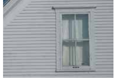
↑ Window casing over clapboard siding. Cookshire-Eaton, Sawyerville sector.
