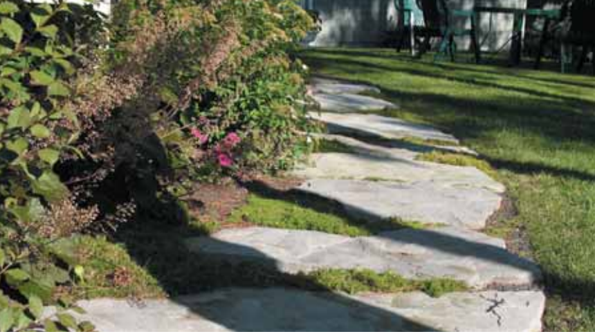
↑ “Stepping stones” made of staggered stones sunk to ground level. Photo: Collection Claude Bergeron
