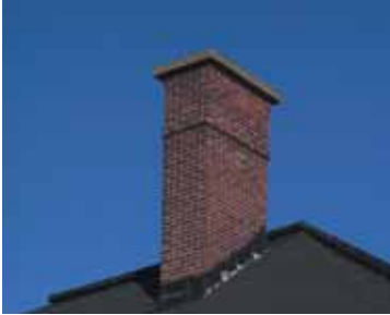
↑ Corbelled chimney, typical of the Victorian period. Dudswell, Marbleton sector.
