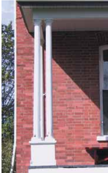
↑ Brick sidings in very good condition. Cookshire-Eaton, Cookshire sector.
