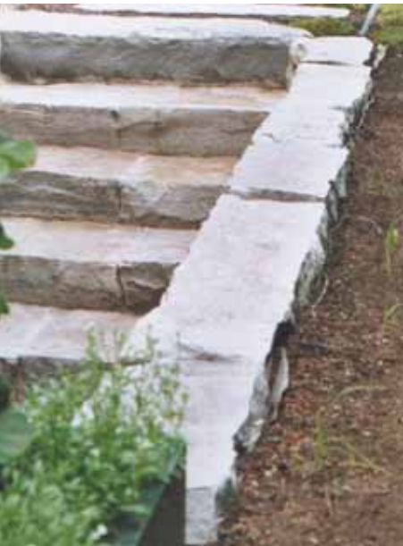
↑ Example of dry stone steps and retaining wall. Photo: Collection Claude Bergeron
